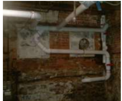
The ladies's room, same perspective, after demolition
